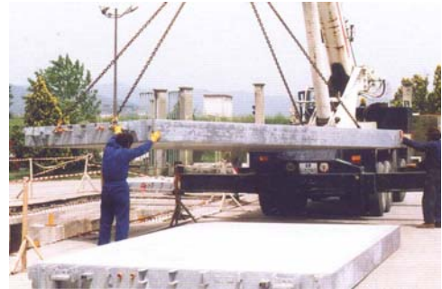
Insertion of the concrete-filled MSBW steel weighbridge modules
