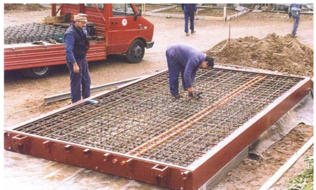
MSBW in-situ concrete solution: Delivery of steel weighbridge frame, on-site concrete
