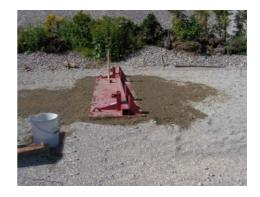
Required ground levelness: 1 cm in relation to the entire mounting length on the longitudinal and transverse plane.
